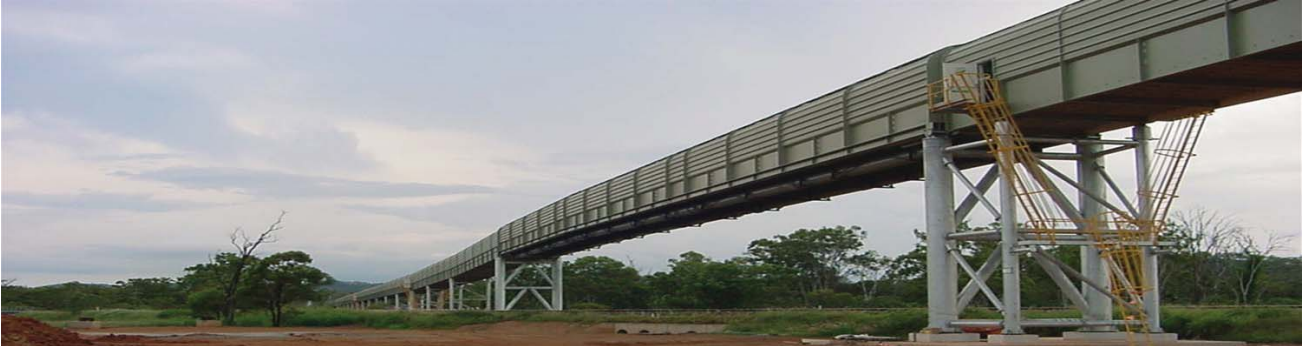
Comalco Alumina Refinery (CAR) – 78 Mtr Span - Enclosed Redispan ® Gallery Conveyor
