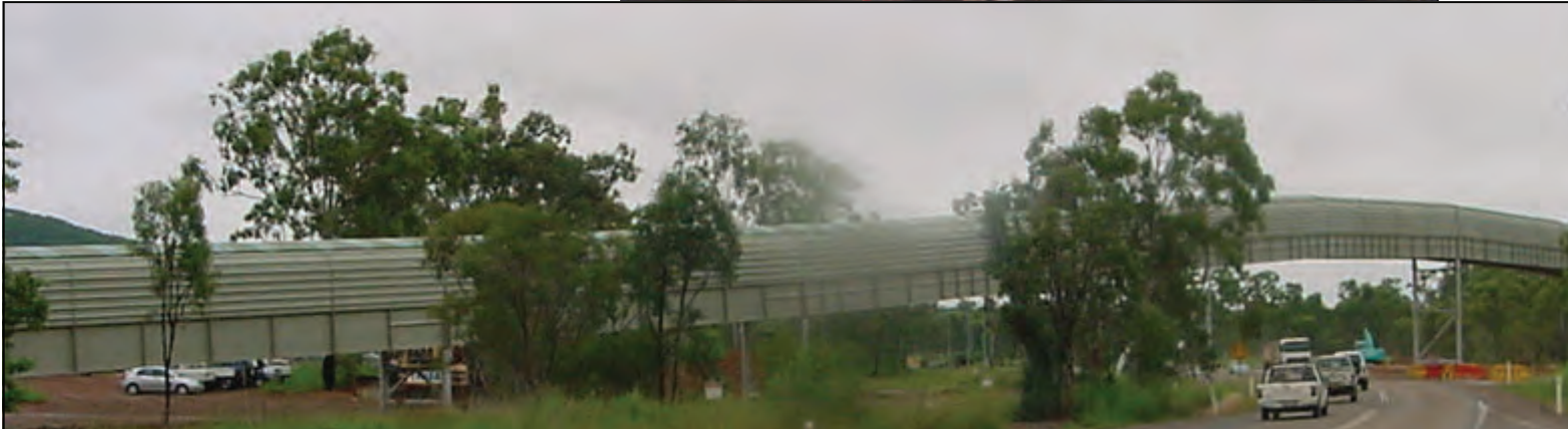
Gantry crossing Bruce Highway
